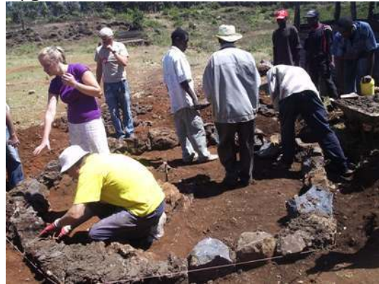
The work team assisting in tank construction in Nkunga School.
