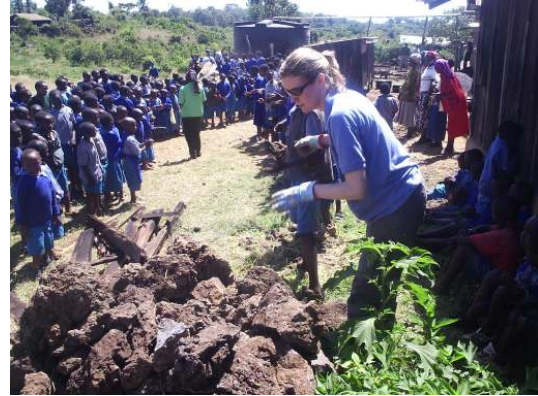
Teamwork and the community collecting hardcore for the kitchen foundation
