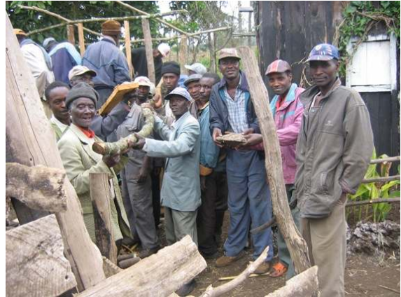
The community participating in the construction of a goat pen.
